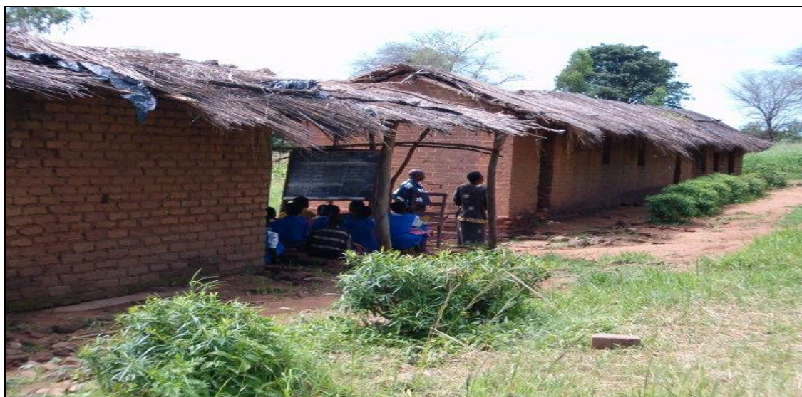
Figure 1: A picture of a rural primary school with poor infrastructure
