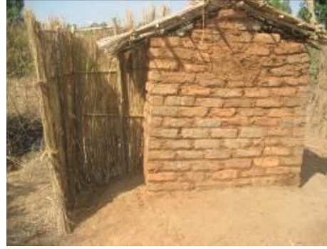
One of the four toilets constructed at Kayuni
